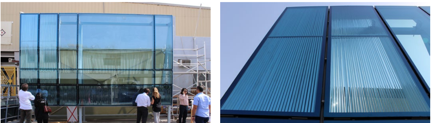
Figure 4. Base Building Curtainwall Modulation: Bay window vision panel flanked by two 750mm vision panels adjacent to vision with micro louver and spandrel.
