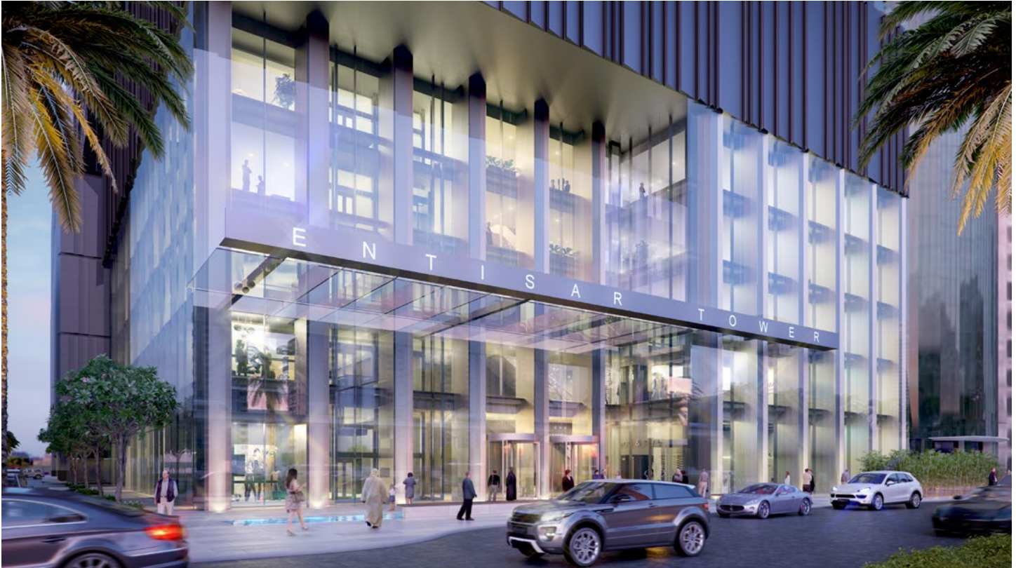
Figure 6. Entisar Tower Podium and Main Entrance. Seventy-Eight foot high double glass skin suspended from mechanical floor
